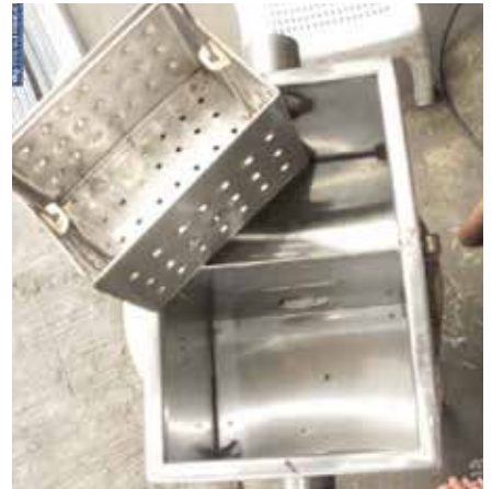
Grease traps have reduced odours and more consistent, less cluttering grease.
