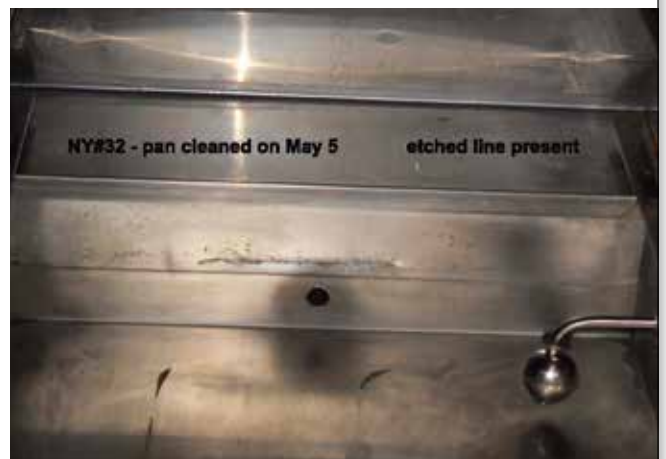
After the installation — pan area is now completely scale-free. There is a slight indentation into the pan at the waterline.
